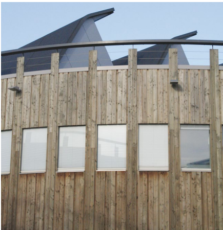
Figure 4: Home-grown larch cladding, Greenwich Millennium School
