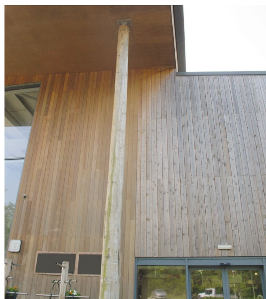
Figure 9: Overhanging roof has protected the wood from weathering
