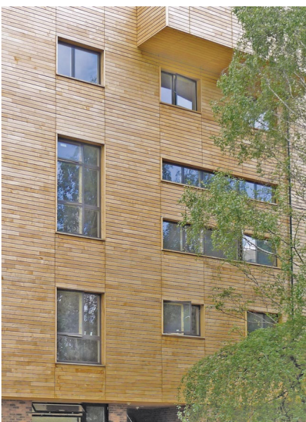
Figure 5: Sweet chestnut cladding, mixed-use building, Whitmore Road, London
