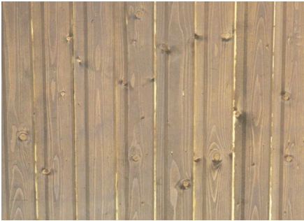
Figure 3: This softwood cladding coated with a stain finish after installation shows the effect of subsequent moisture movement
